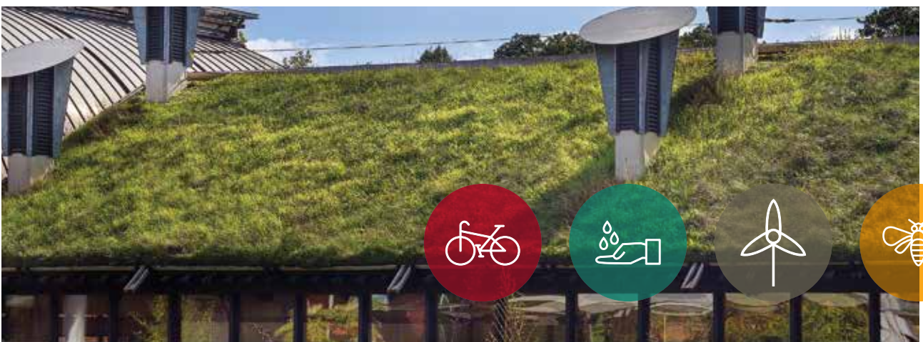
Figure 5: Further example of a green roof
